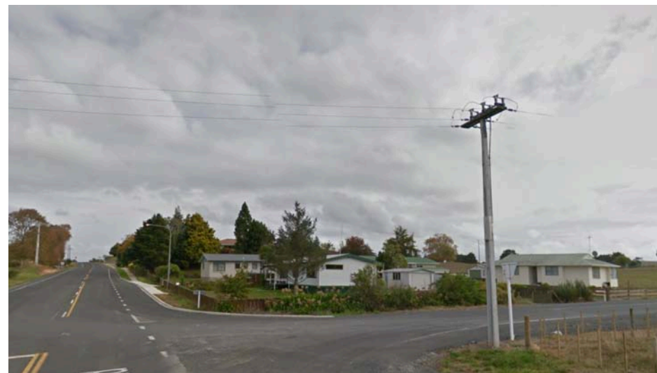
Intersection of Waerenga Road and Swan Road looking west
