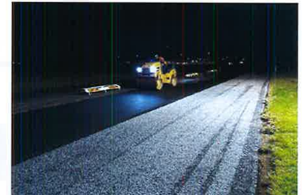
Asphalt being laid to defective area - Taxiway 'D'
