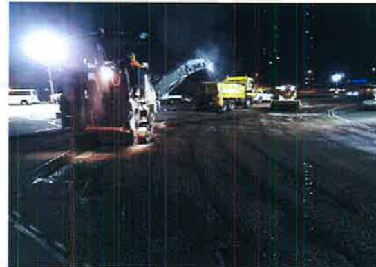
Milling of Intersection of RWY 18L/36R and Taxiway 'A'
