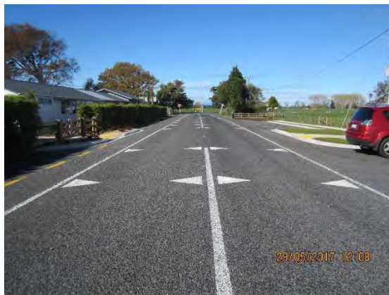
Sainsbury Road Rehab where the WDA capitals works team were recognized for their exceptional work in reducing a significant risk to school children
