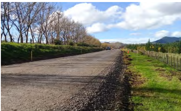
McVie Road Rehab
