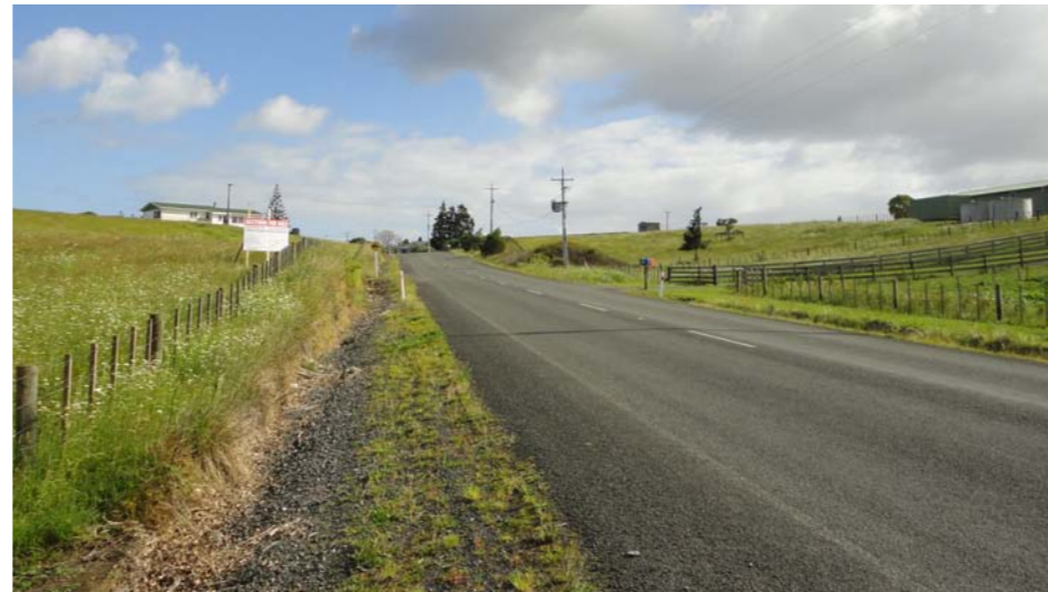
View north on Swan Road depicting space available for shared path
