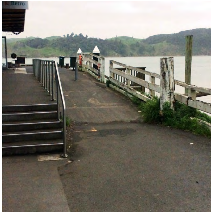
Image 1 – Raglan Wharf handrail
