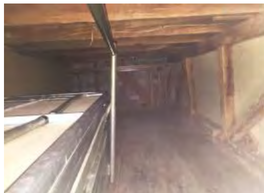
Timber trusses and floor joists supporting the stage deck
