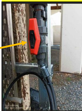
Incorrect location valve and hose detached by sampler 4 (IP)
