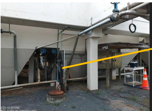
Incorrect location valve and hose detached by sampler 4 (IP)
