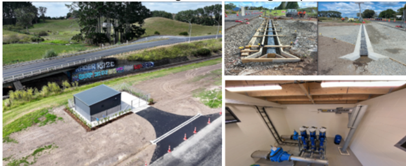
Taupiri Water Supply Booster Pumpstation is nearing completion.
