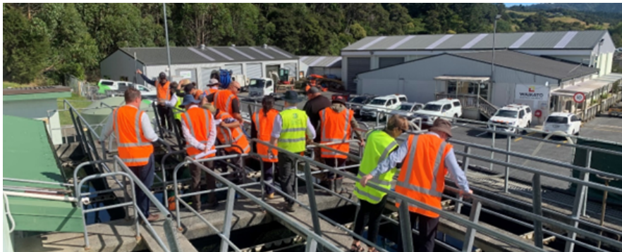
Figure 2: Site visit with mana whenua to the Ngaaruawaahia Water Treatment Plant.
