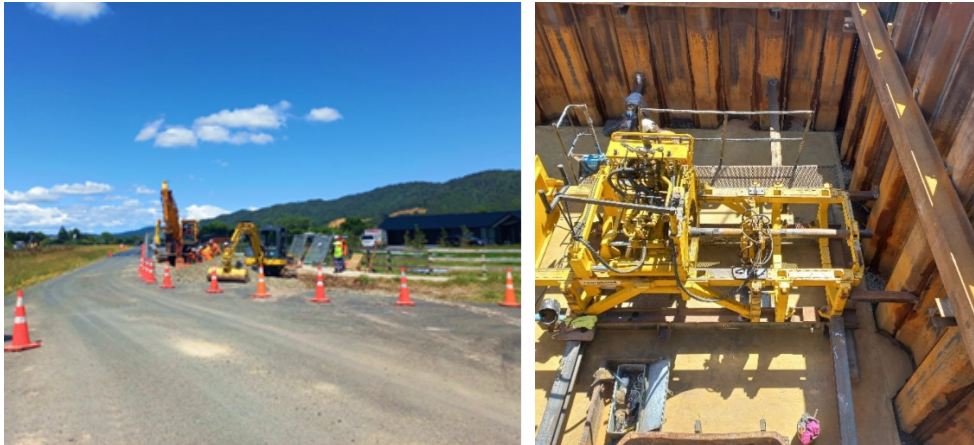
Ngāruawāhia Pipeline - Galbraith St works and the undertrack auger pilot bore
