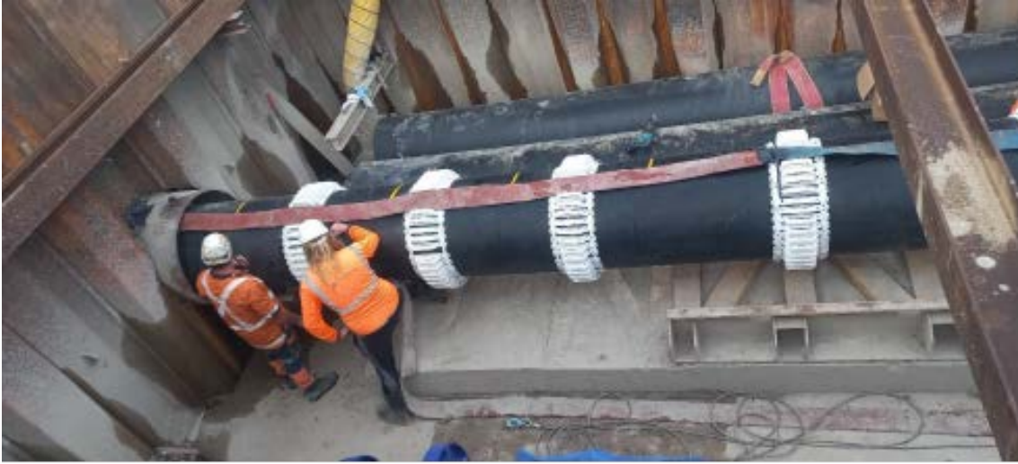
Ngaaruawaahia Pipeline - The undertrack pipe being pulled into the casing
