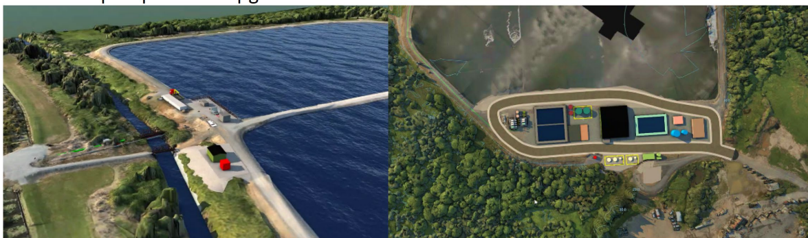
Huntly WWTP Upgrade Concept Design: New outfall Pump Station and the future MBR Upgrade
