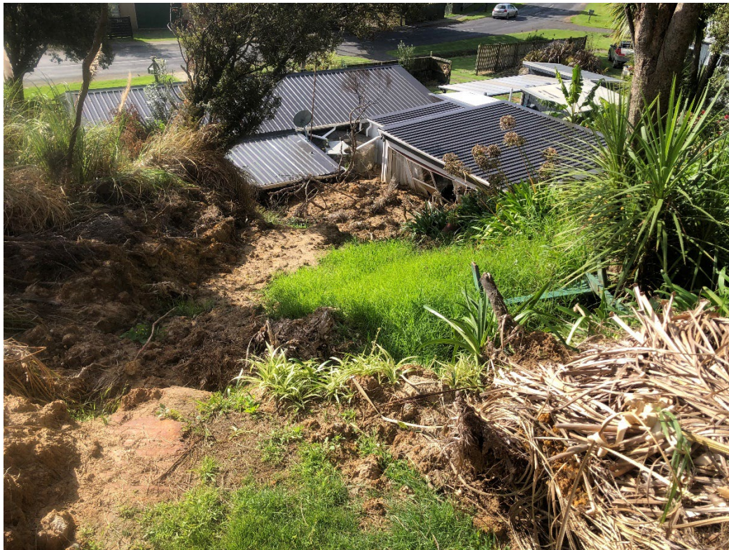
Photograph 6: View looking north from behind dwelling at 159 Maunsell Road (Landslide 12)
