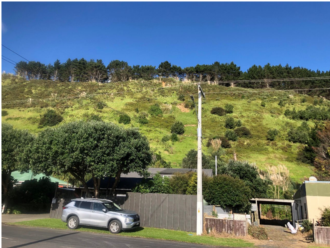
Photograph 10: Landslide above 123 Maunsell Road
