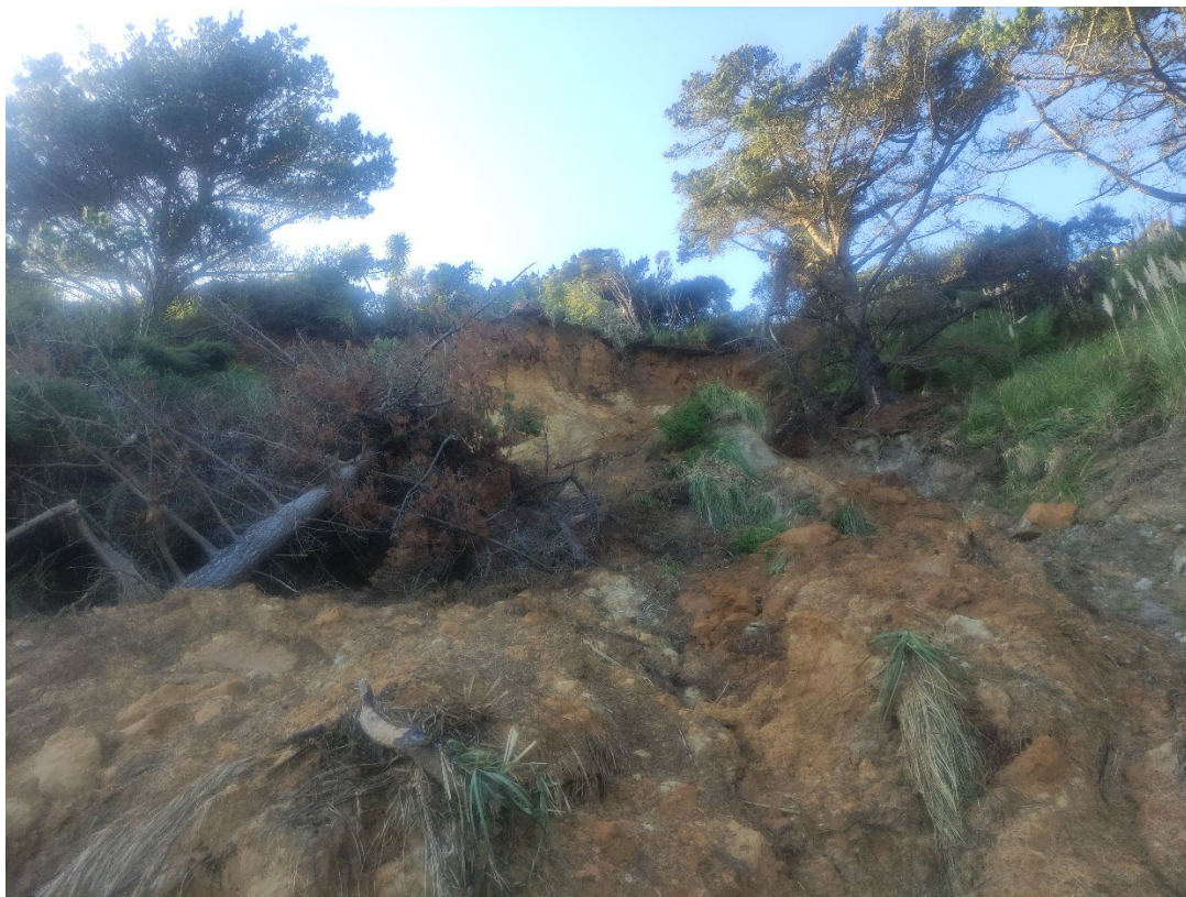
Photograph 4: View of Landslide 5 above 201 / 199 Maunsell Road
