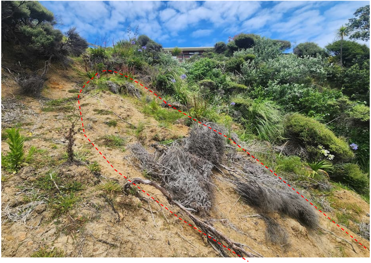
Photograph Appendix B.5: Landslide 2A
