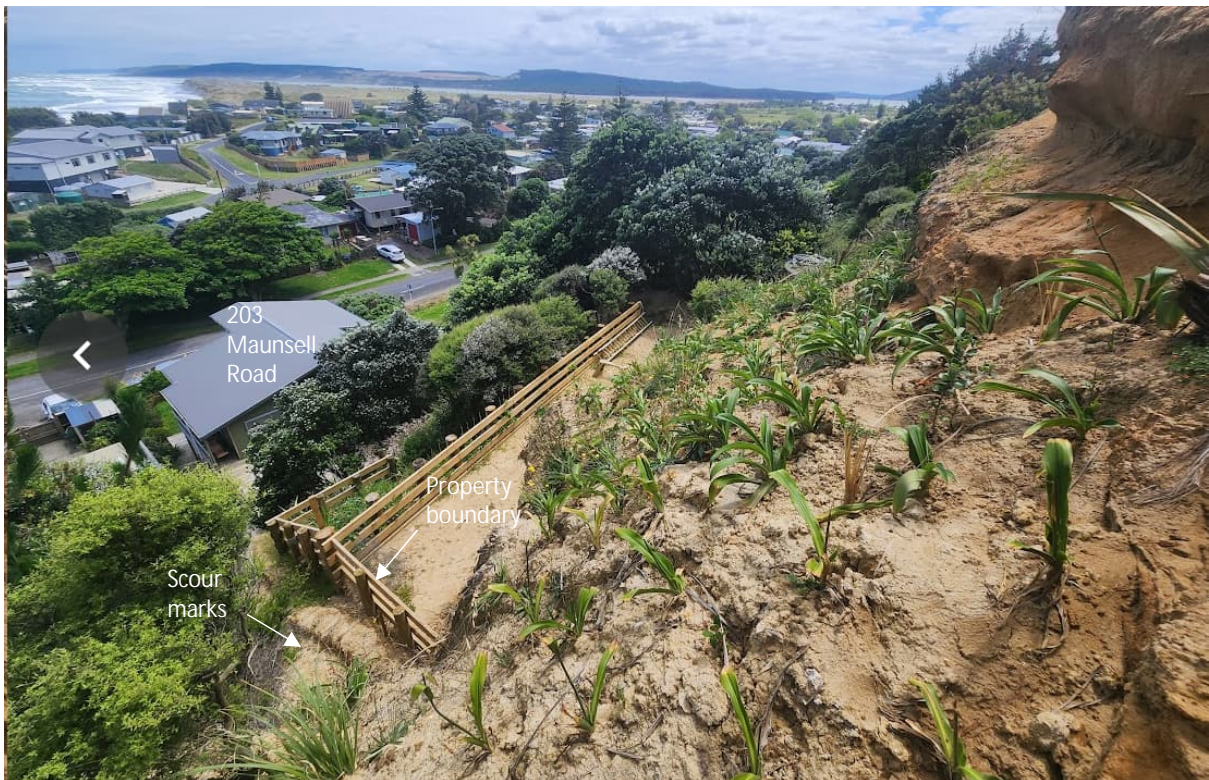
Photograph Appendix B.10: Landslide 1
