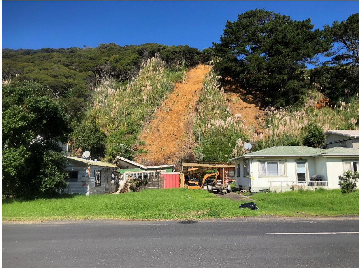
Photograph 5: View of landslide 9 above 175 and 177 Maunsell Road
