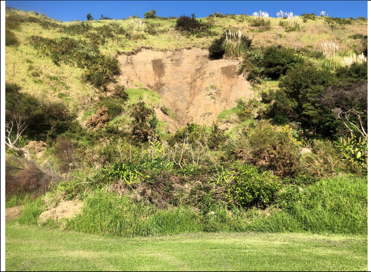
Photograph 1: Port Waikato Holiday Park, Large Landslide 19
