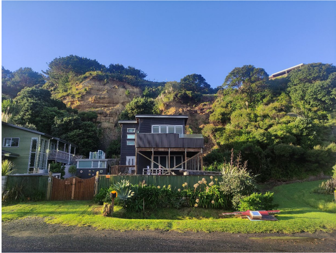
Photograph 3: View of Landslide 1 & 4 from northern side of 205 Maunsell Road
