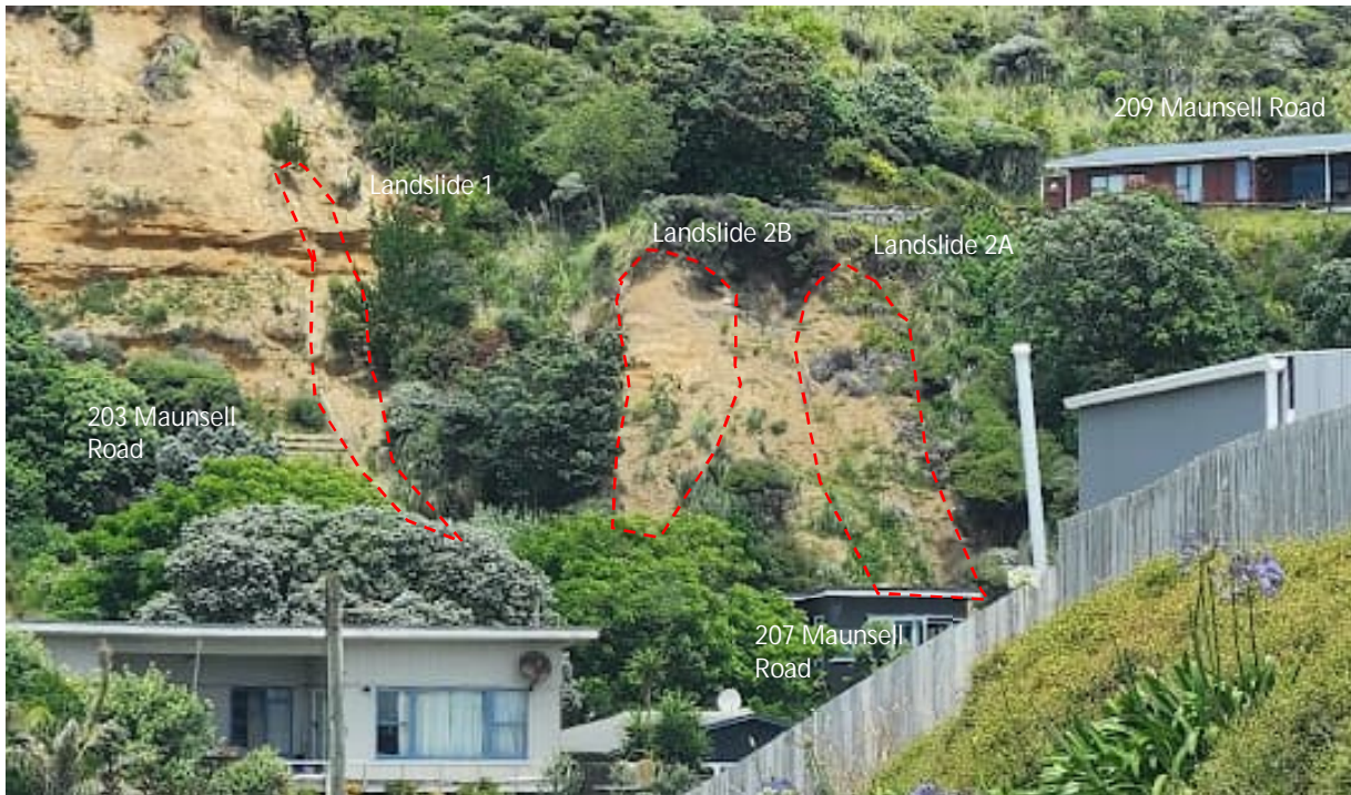
Photograph Appendix B.1: Site overview
