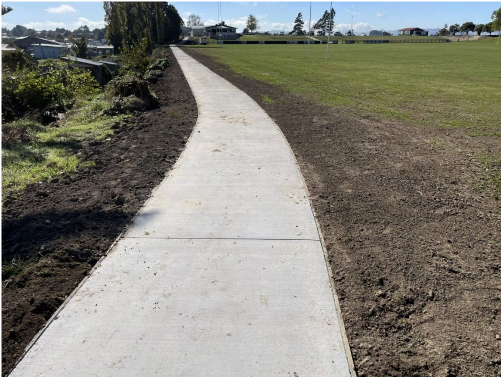
Concrete path construction
