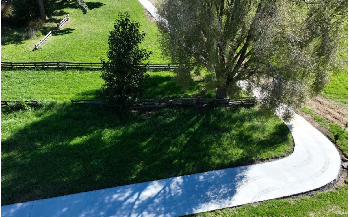
Concrete path construction
