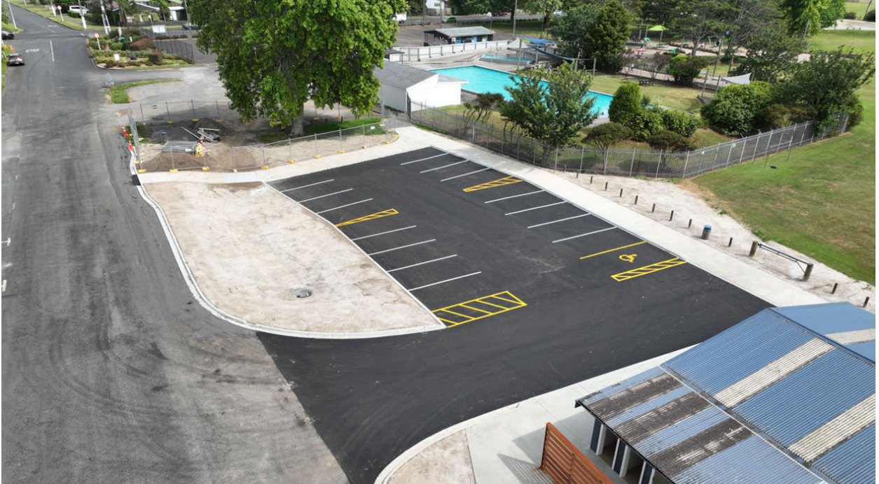
Southern carpark complete.
