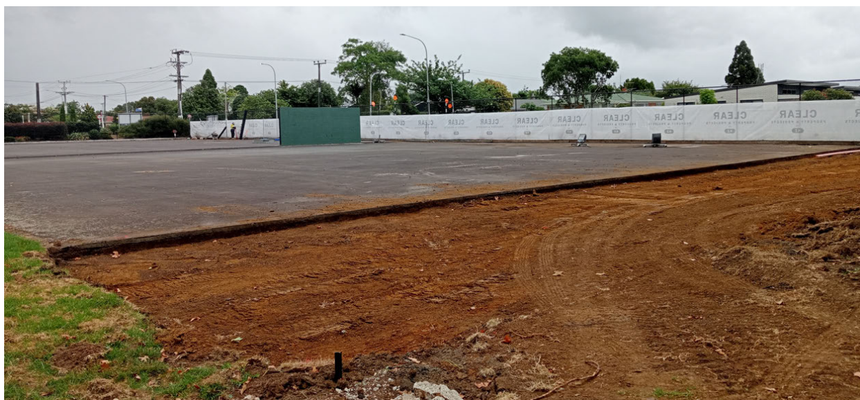
Work underway on the courts.
