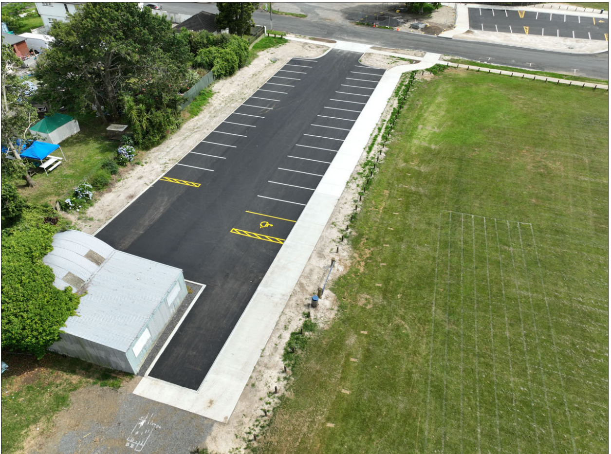
Western carpark complete.
