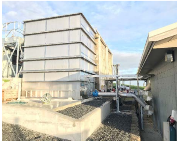
New BAC Filter Te Kauwhata WTP
