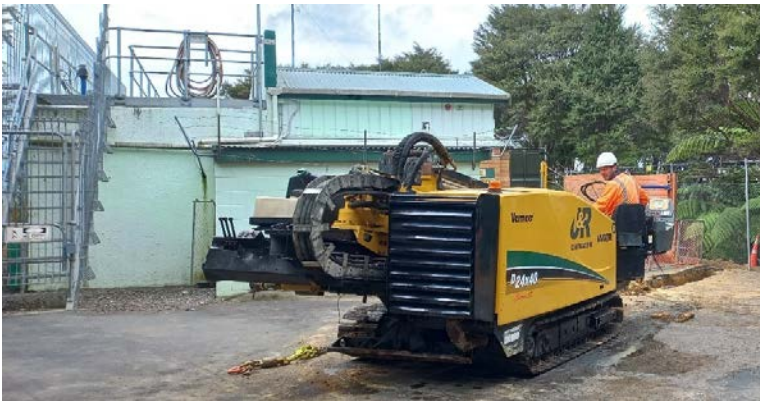
Ngaruawahia WTP Upgrade – Run to waste horizontal directional drill installation
