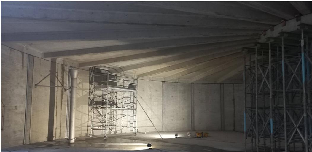
*Te Kauwhata Reservoir 1 - Roof complete, joint sealing underway*
