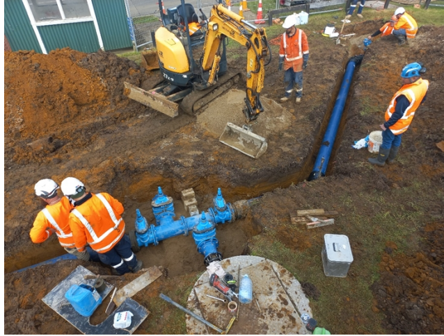
Raglan – One of seven critical tie-in points
