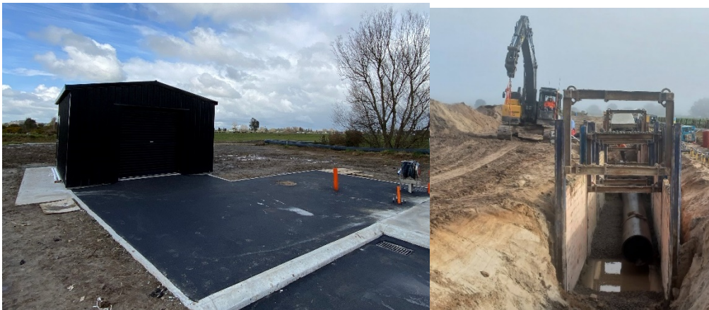
Ngāruawāhia Pipeline – New Inlet Pump Station and continued pipeline construction
