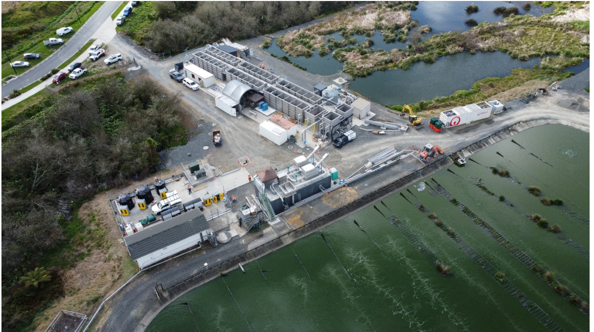
Te Kauwhata WWTP – Construction fit-out underway
