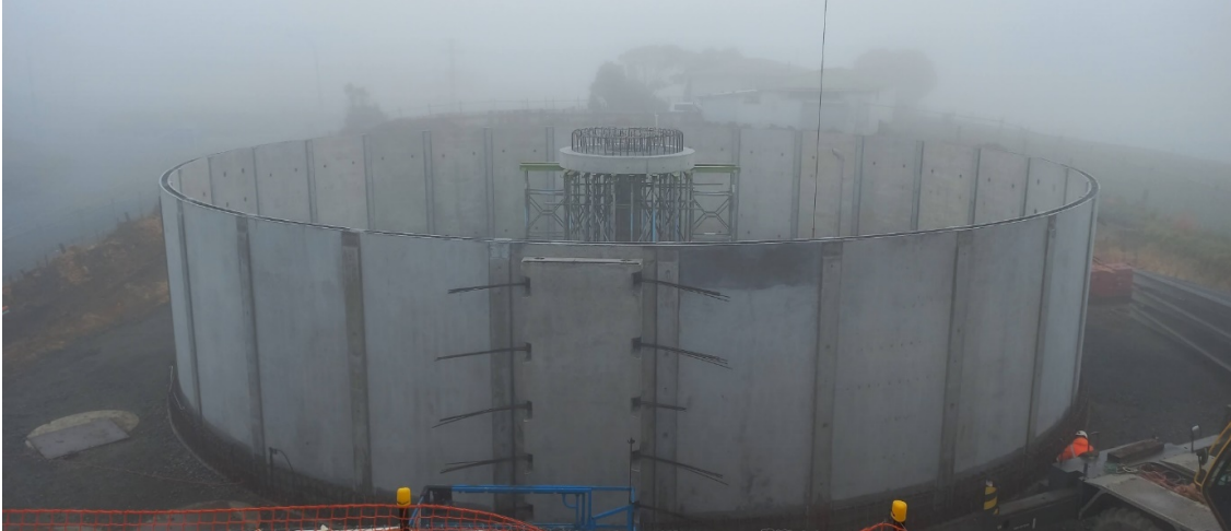
Te Kauwhata – Reservoir 1 – Post tension super strand awaiting grout and capping
