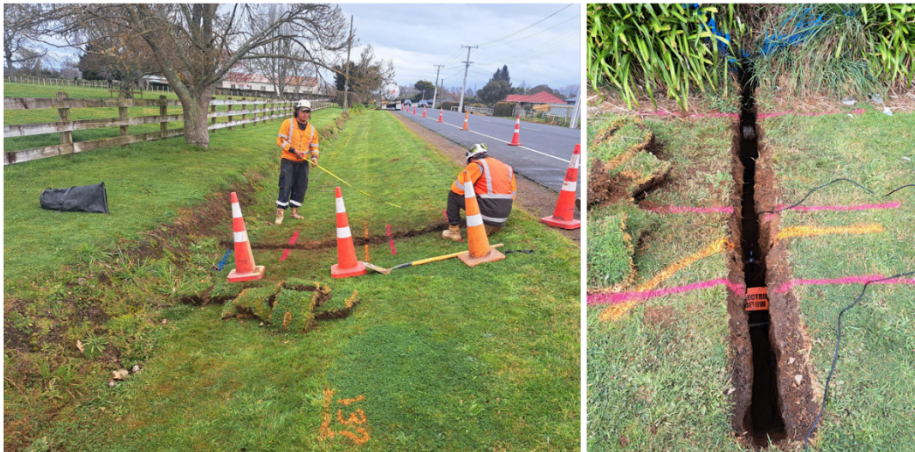
Morrinsville Road – Utility mapping/design confirmation underway
