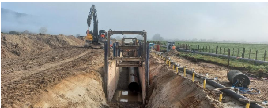
Ngāruawāhia Pipeline – Construction supported by well-pointing at the second farm crossing
