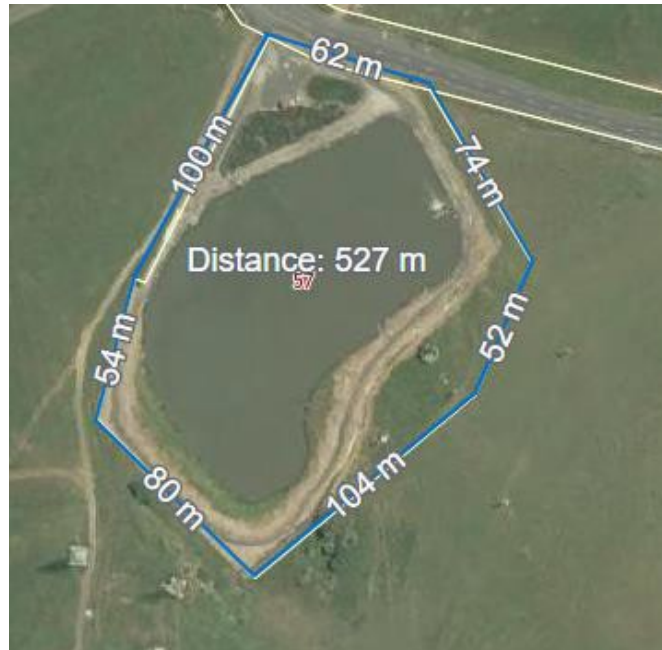
The Meremere wastewater treatment
