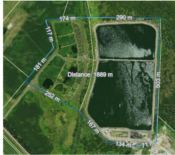
Te Kauwhata wastewater (ponds and wetland),
