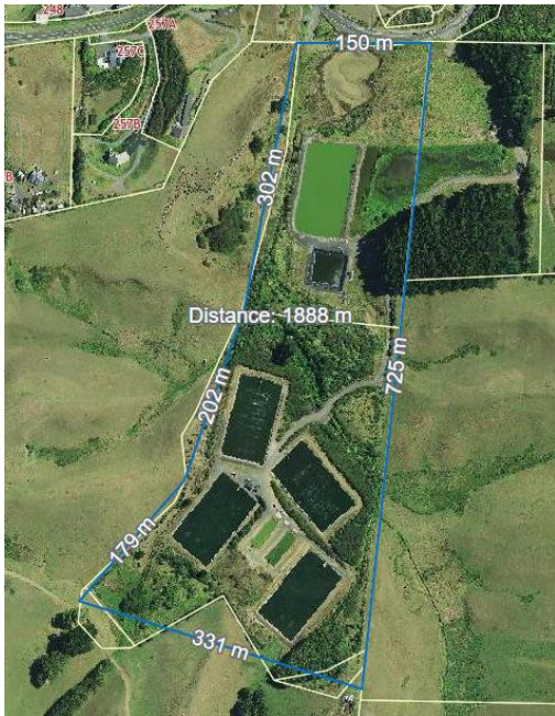
Raglan waste (ponds and wetland)
