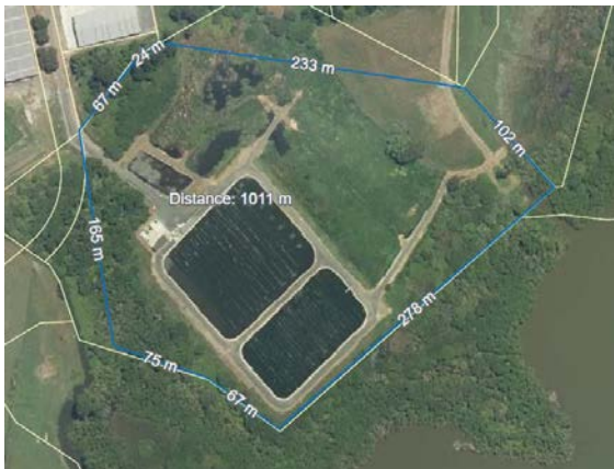
Te Kauwhata wastewater (ponds and wetland),
