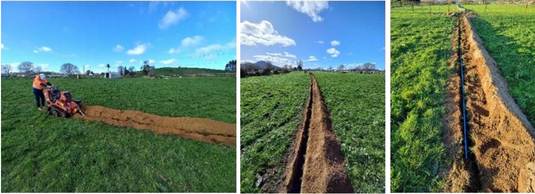
Taupiri – water main installed via chain trencher
