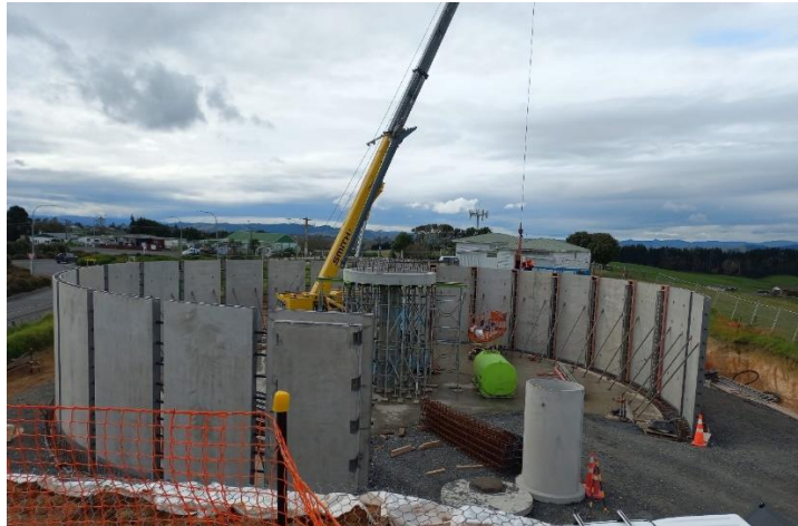
Te Kauwhata – Reservoir 1 – Floor slab main concrete pour
