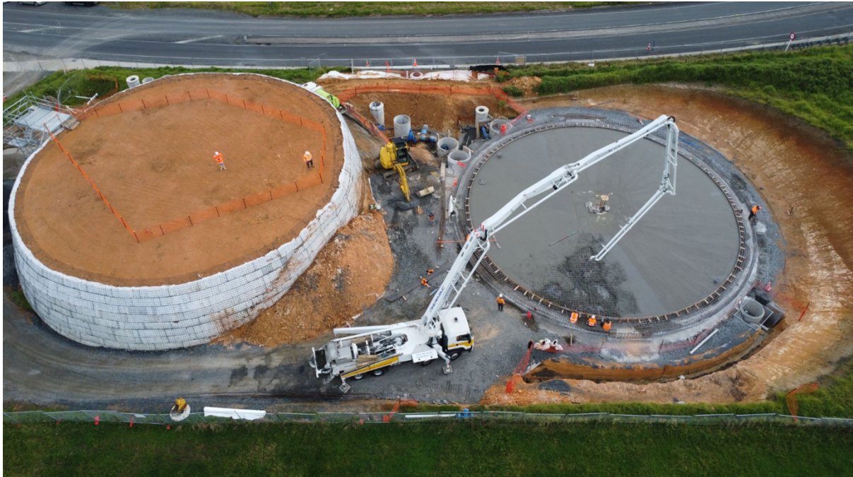
Te Kauwhata – Reservoir 1 – Floor slab main concrete pour
