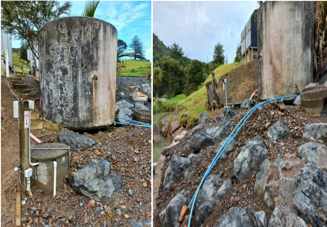
Port Waikato Water treatment plant – bank reconstruction.
