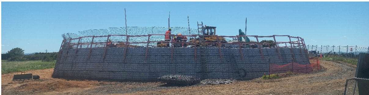
Te Kauwhata – Reservoir 2 preload construction
