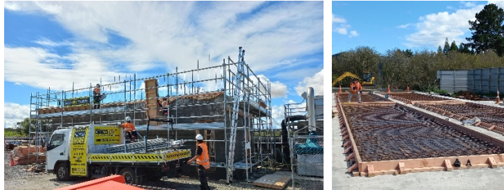
Te Kauwhata WWTP – New Blower room and MABR tank upstand construction
