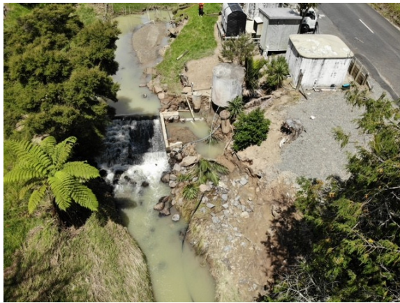
Port Waikato water treatment plant damage to stream banks
