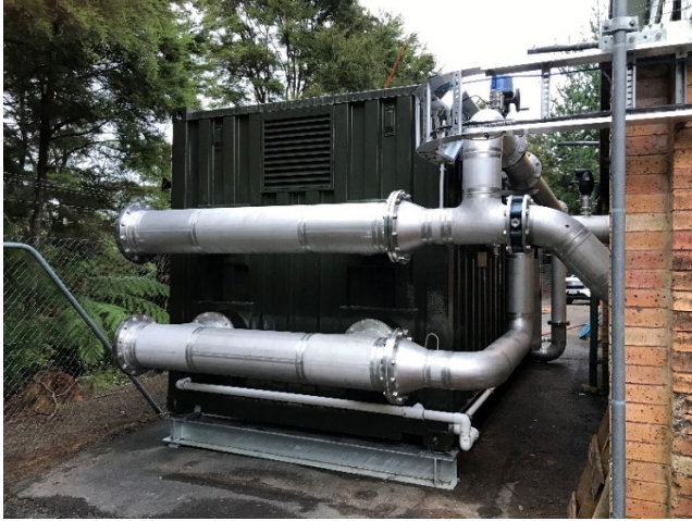
Ngaruawahia UV treatment units and connection pipework
