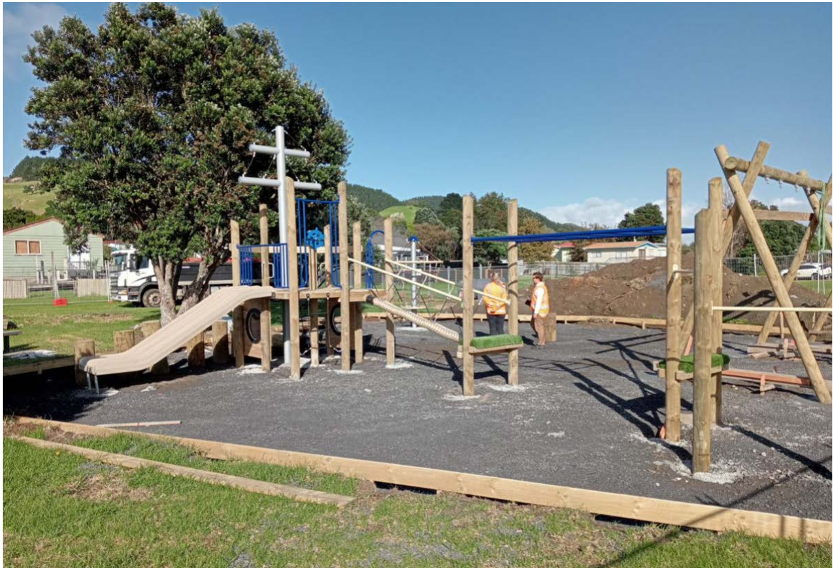
Maraetai Bay Playground construction
