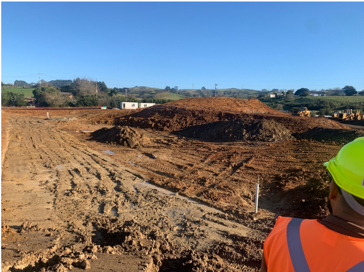
Earthworks is currently on hold due to the wet weather
