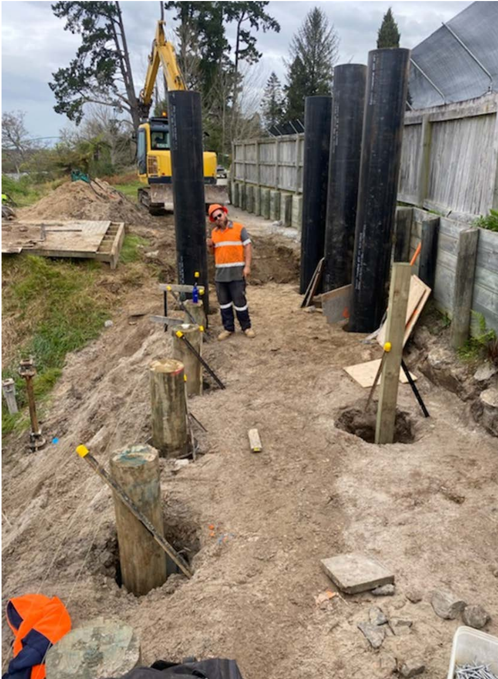
Timber piles and steel pile casings being installed.
