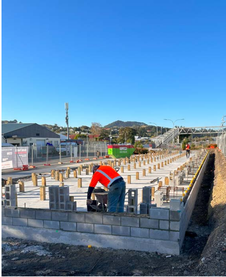
Block work in progress and poured concrete foundation
