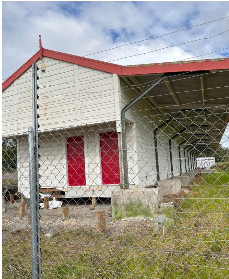
Building preparation works - Decking removed ready for concrete pile removal.
