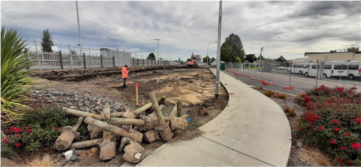
Clearing the site for foundation works
