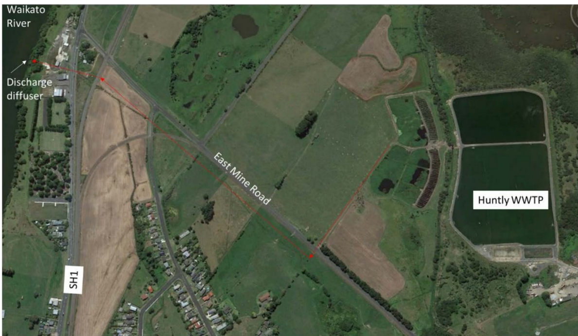
Aerial photos of the Huntly WWTP and surrounds
