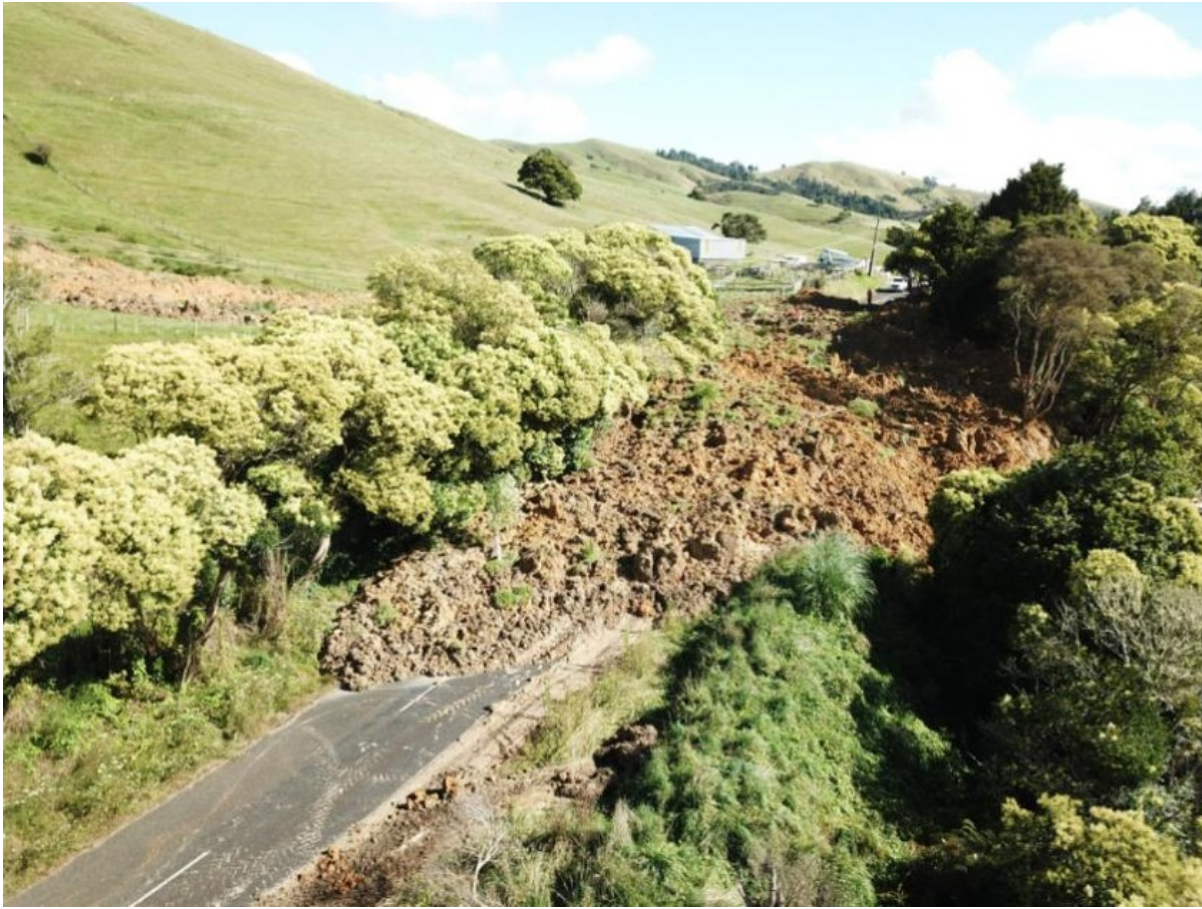
Matahuru road slip, very large volume of material that required moving
