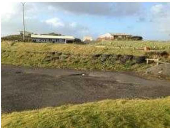
Photograph 4: The lower car park with tyre retaining wall at the rear.
