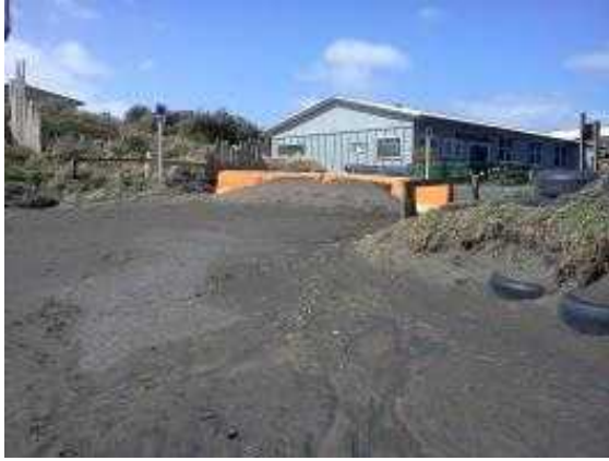
Photograph 8: Sand being deposited against temporary concrete barriers in the middle of the upper and lower car park, northern end. Looking east toward the community hall.
