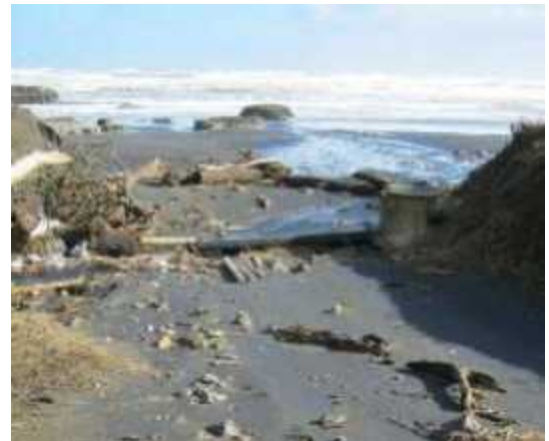
Photograph 13: Photo from 2011 showing connecting pipe that has been removed.
