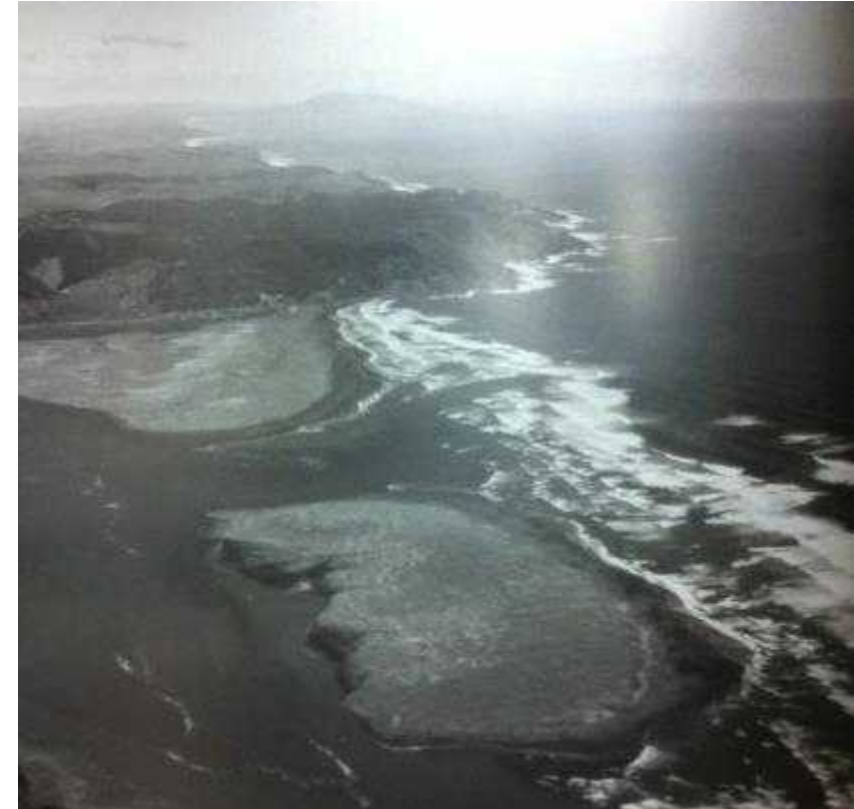
Figure 4: Spit Breach in October 1960 (Source: Port Waikato Dairy)
