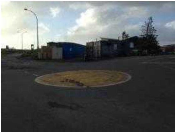
Photograph 10: Large area of paving currently used for road roundabout that could be more efficiently utilised. Recycling facilities behind round about.
