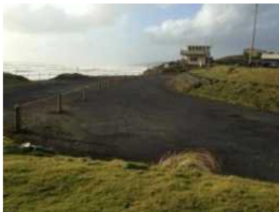
Photograph 5: Lower car park (looking north) with tyre retaining wall to the right of the photo.
