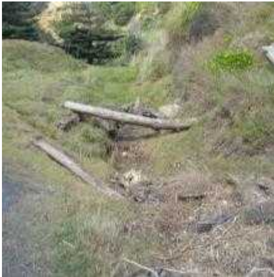
Photograph 11: Natural stream at the base of the southern cliffs looking east, blocked with debris.
