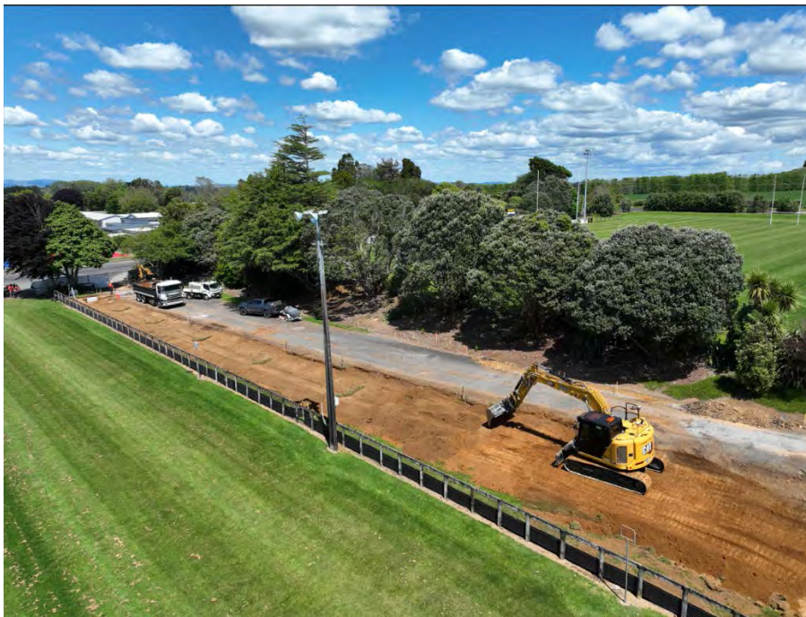
Earthworks at accessway
