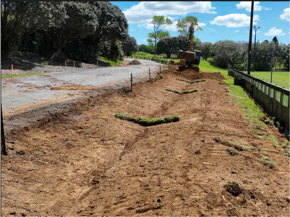
Swale being formed
