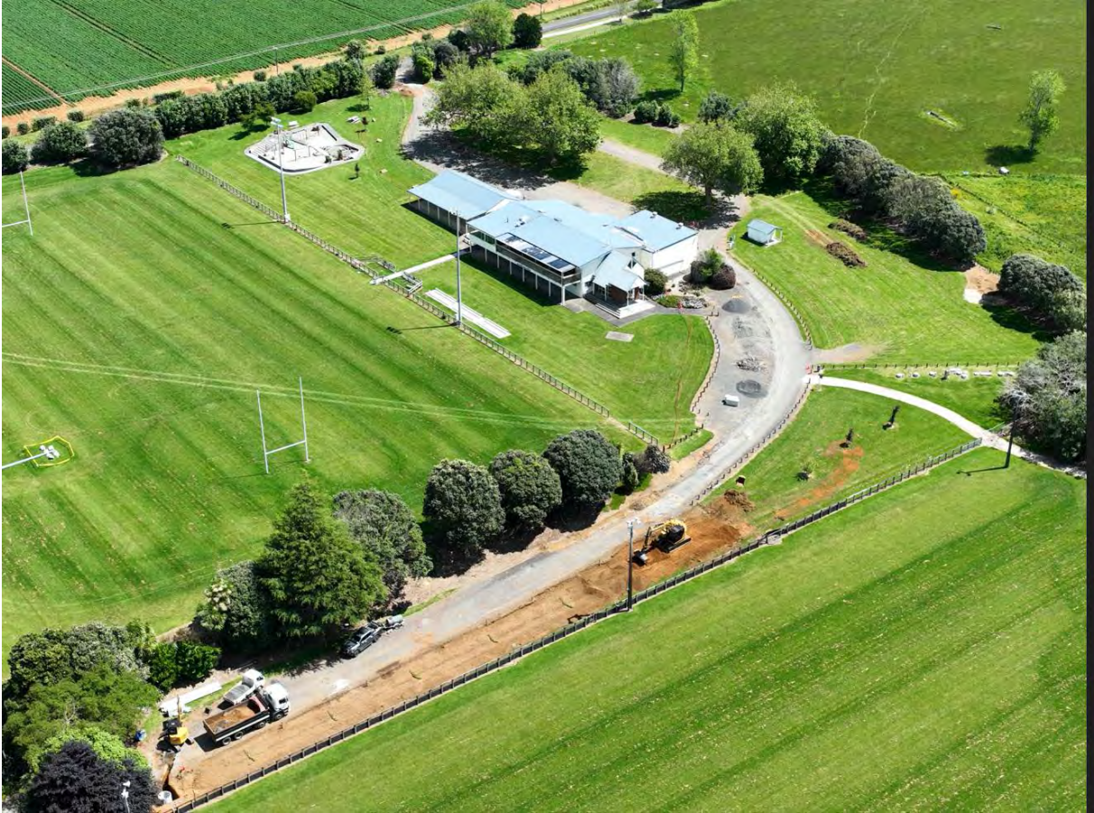
Onewhero Domain Carpark Upgrade – stormwater work underway
