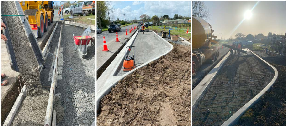
Te Kauwhata Filling Station – Under Construction
