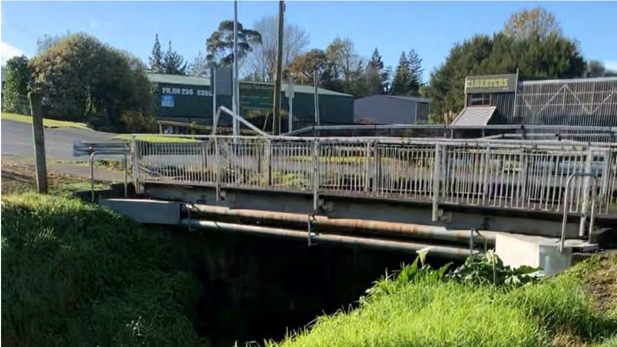
Harrisville Bridge – note service ducts attached to the pedestrian bridge.
