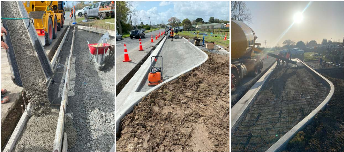
Te Kauwhata Filling Station – Under Construction
