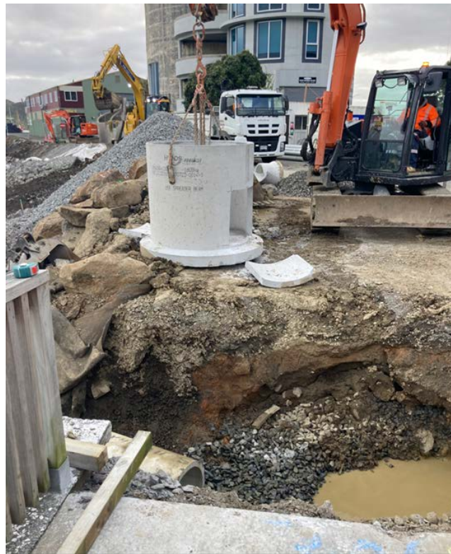
Drainage works with manhole going in.
