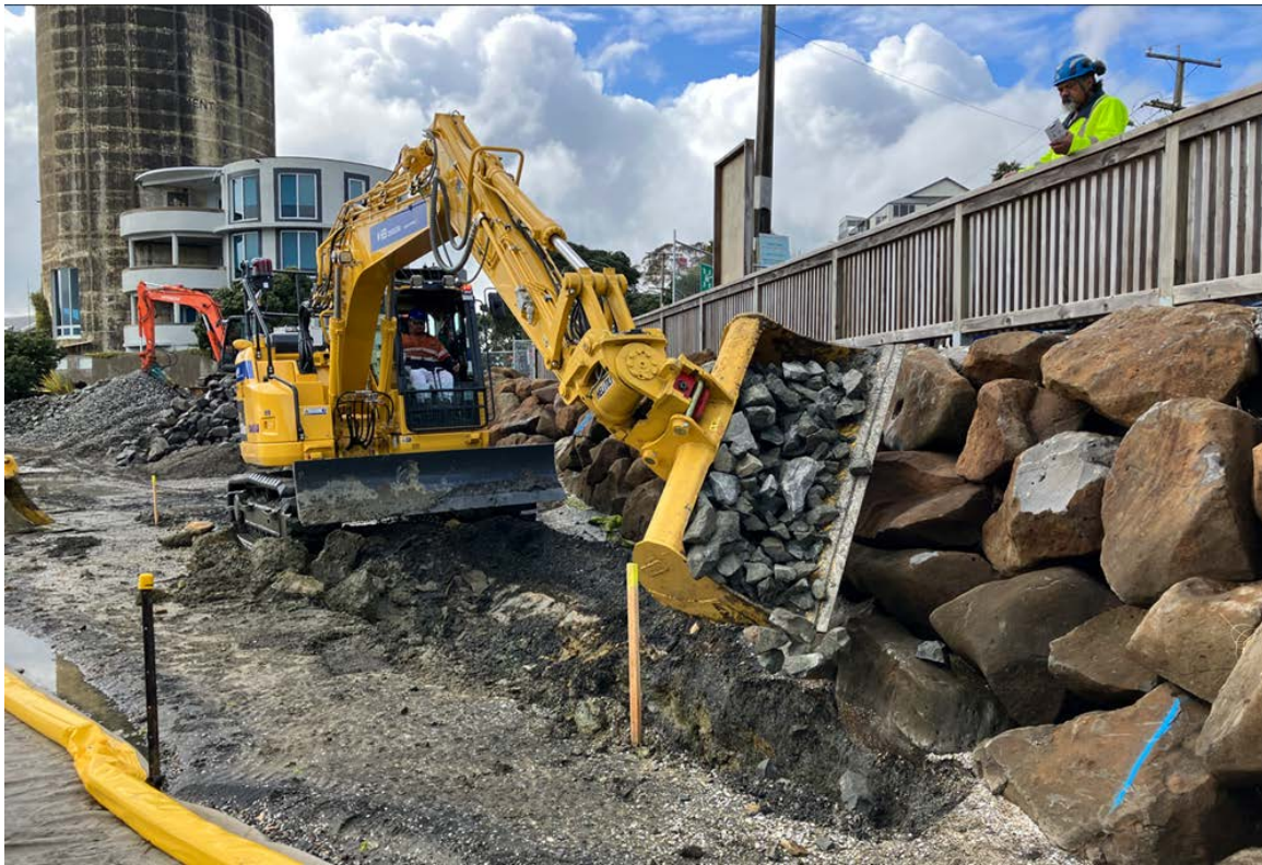
Creating a hold for the toe boulders
