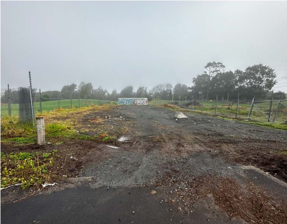
Secure compound to have concrete removed, surface levels, and fence reinstated.
