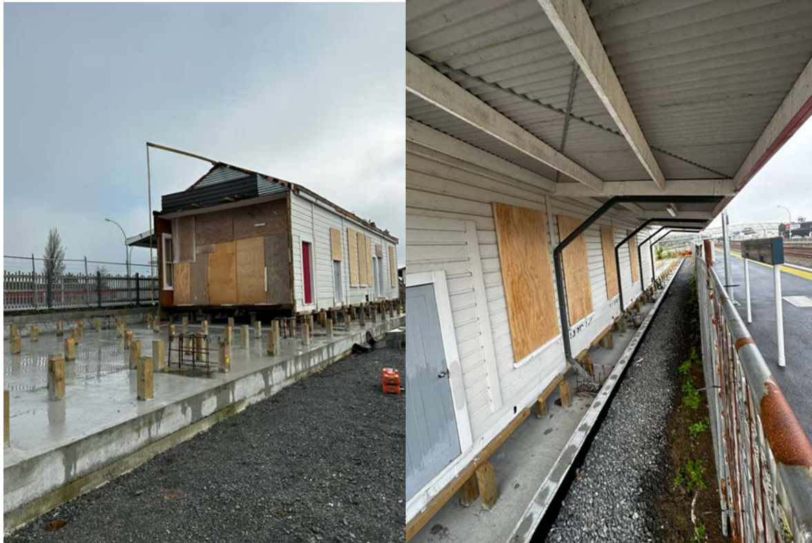
Plywood attached for protection of windows
