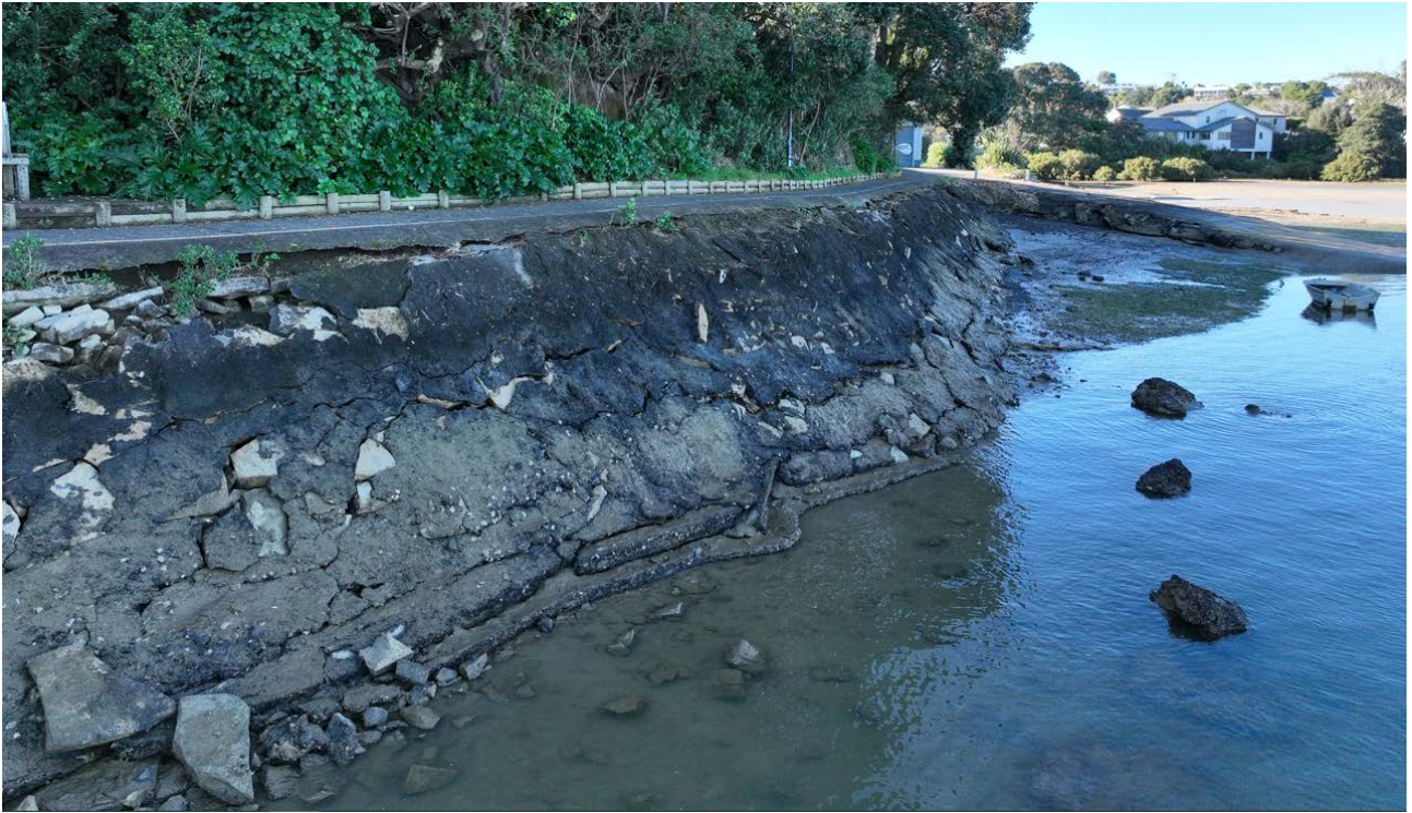
South of the footbridge
