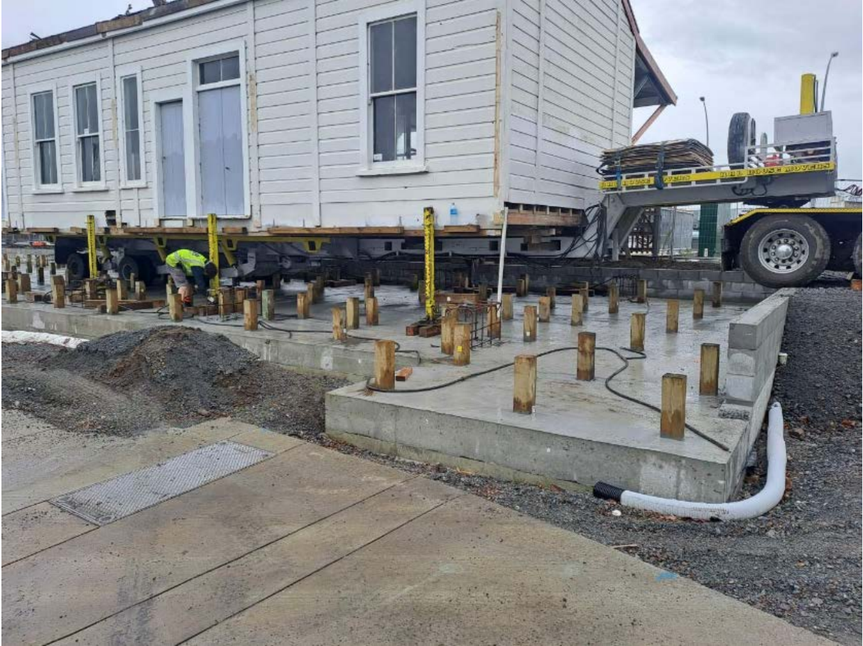
Second section being placed on its permanent foundations.
