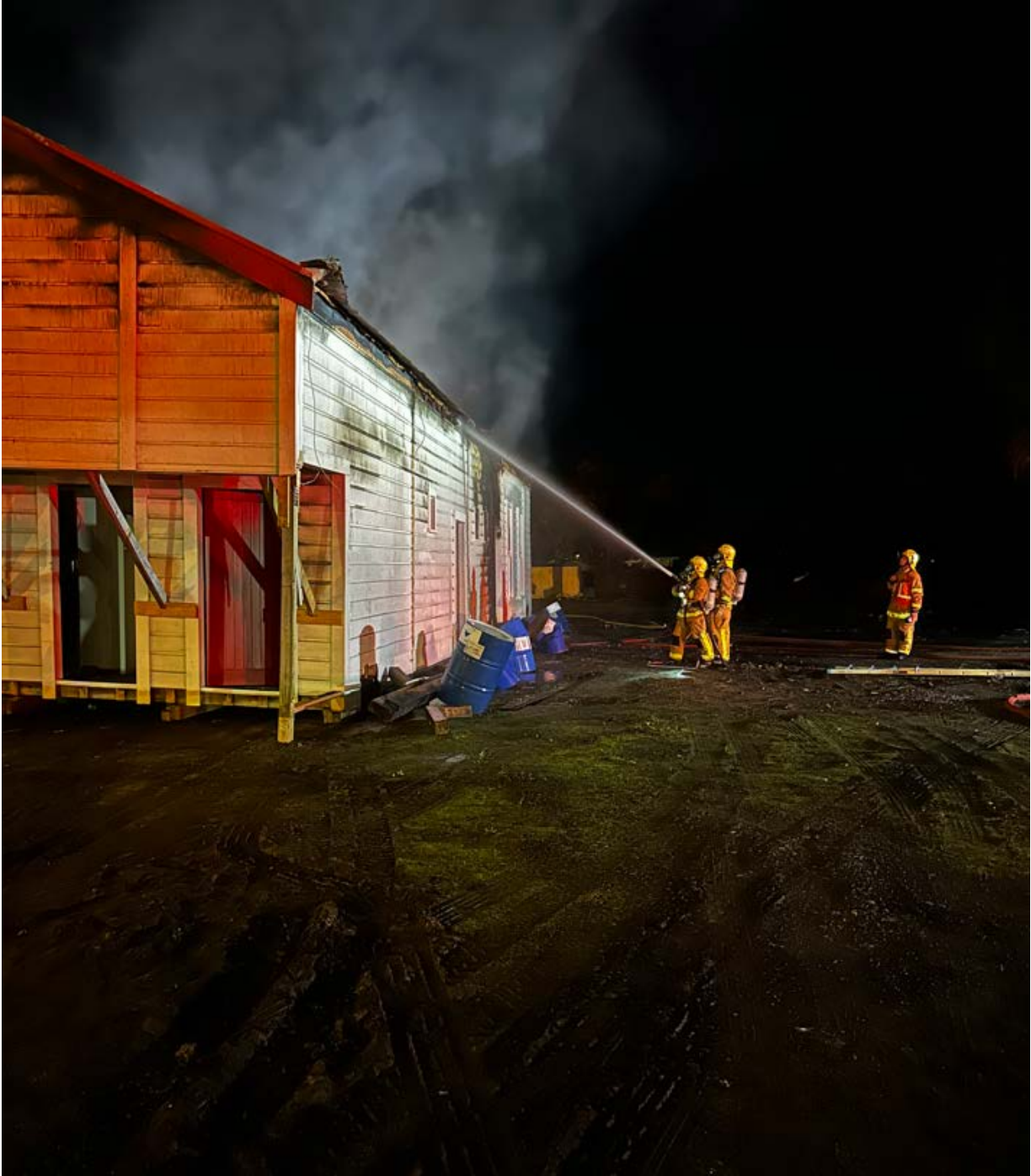
First section on fire during the relocation of the second section of the building.
