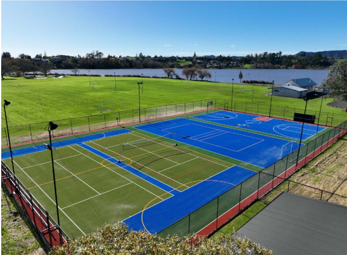
Completed Huntly Tennis Courts
