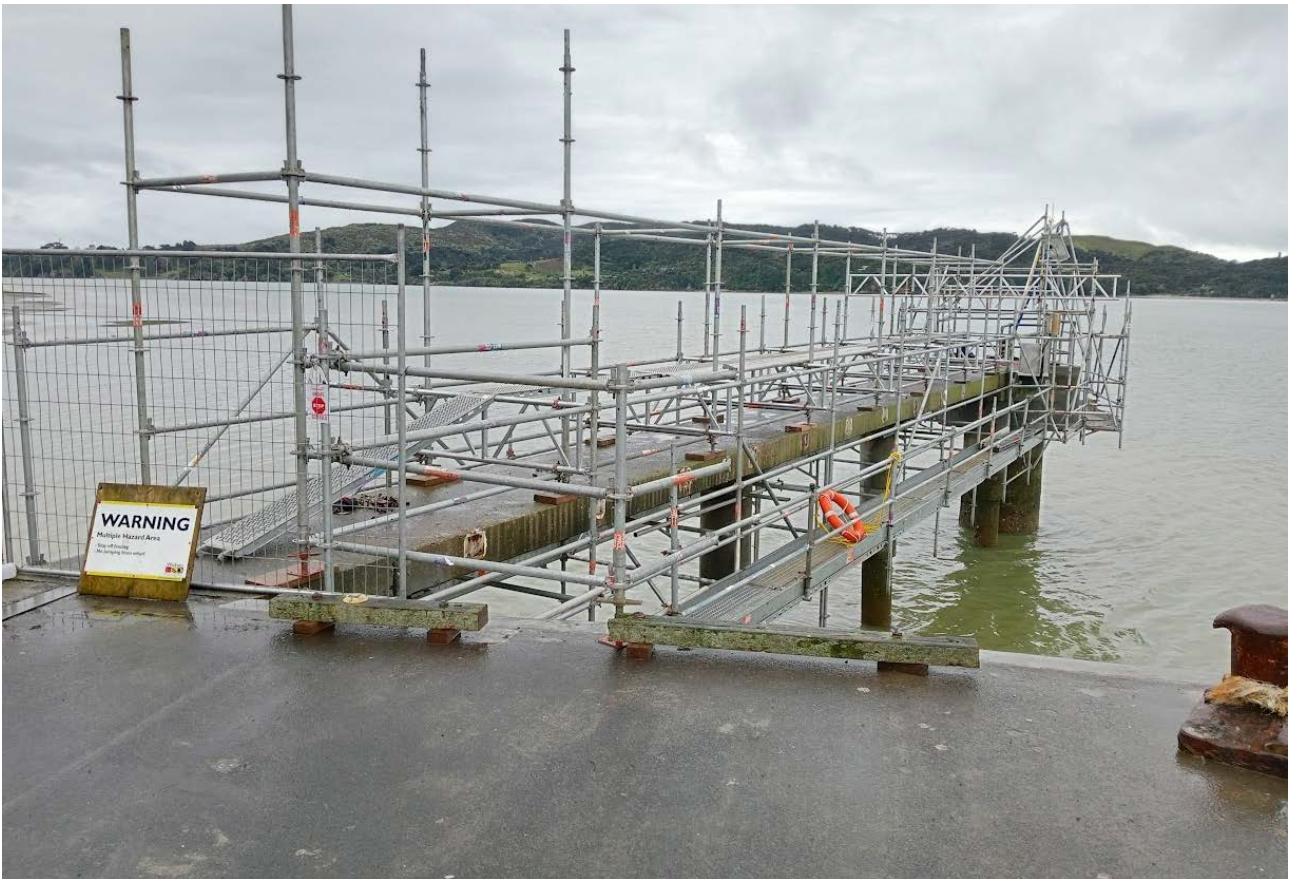
Scaffolding in place for balustrade installation
