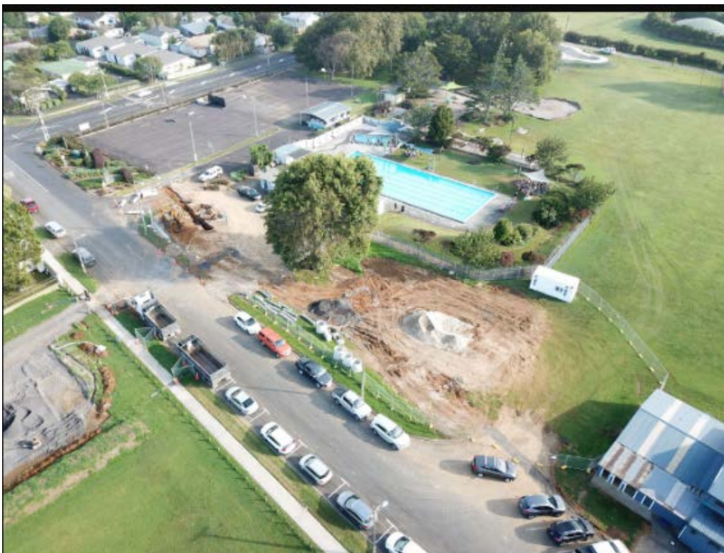
Carpark construction adjacent to the Aquatic Centre
