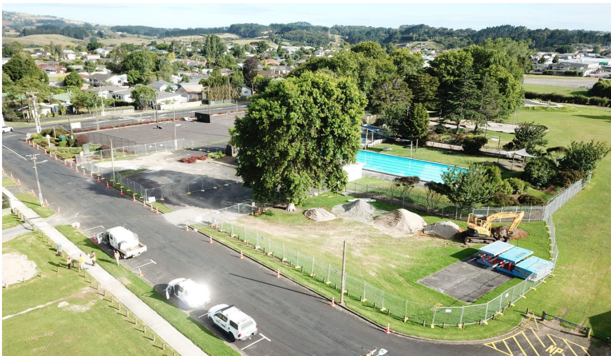
View of the carpark construction looking northeast
