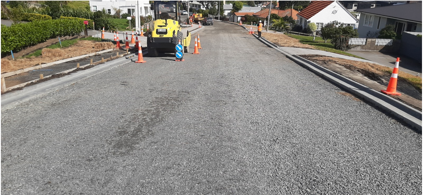
Looking South down Gilmour Street
