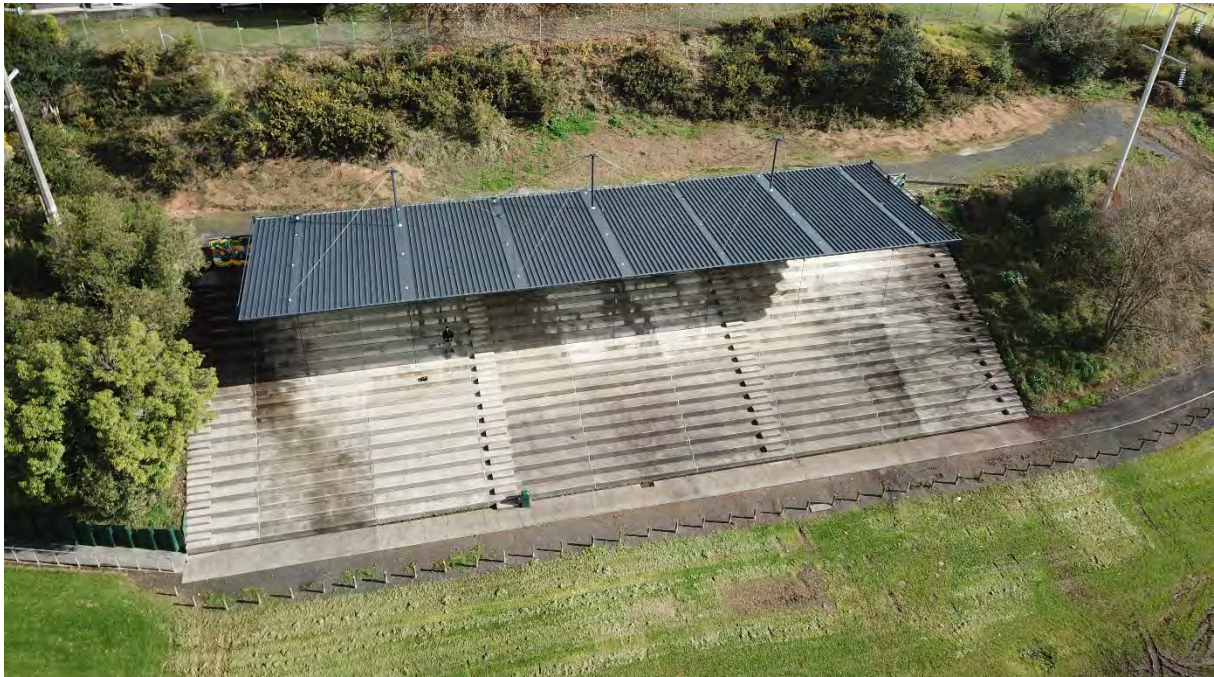
Huntly Grandstand Roof completed
