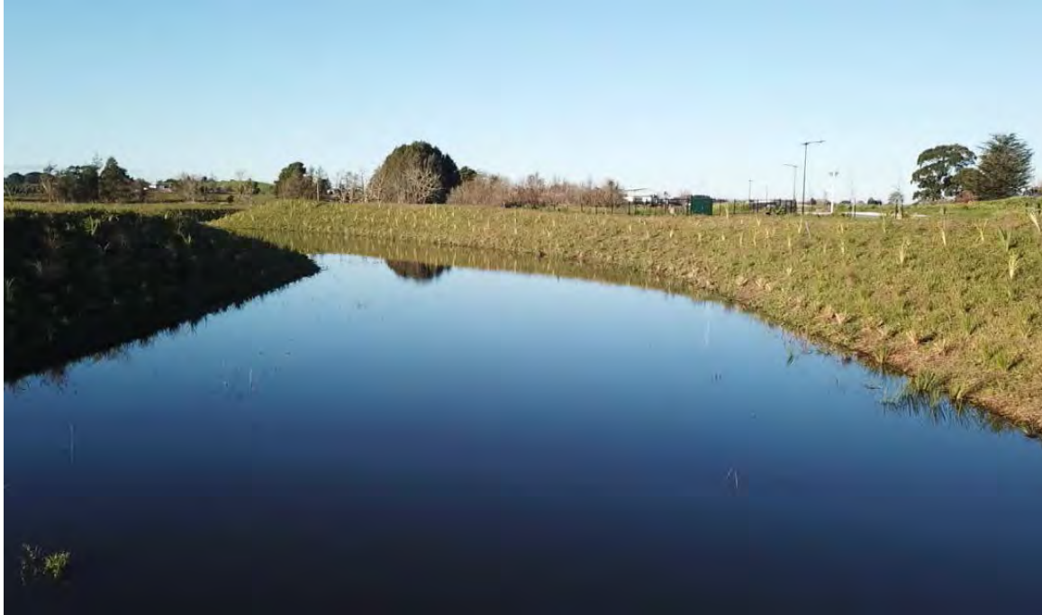
Planting of the new stream alignment is complete.
