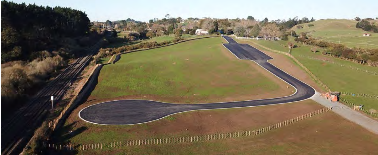
Asphalt is complete on the access road. Vegetation is establishing.
