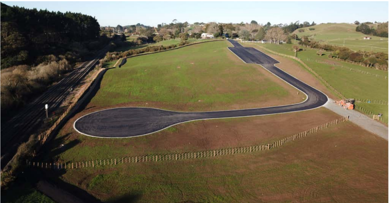
Asphalting of the accessway surface completed.
