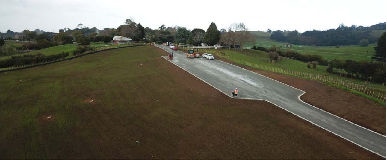
Kerbing and pavement finishing.
