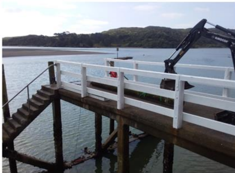
Fender Pole Replacement Underway
