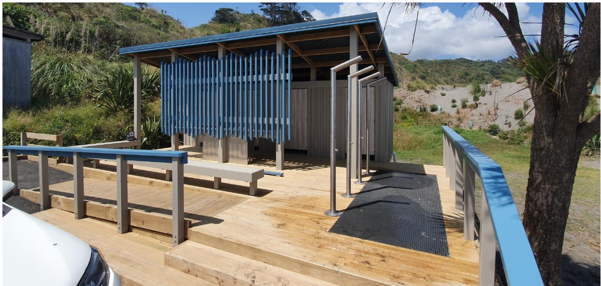
Completed toilet and outdoor shower facilities.
