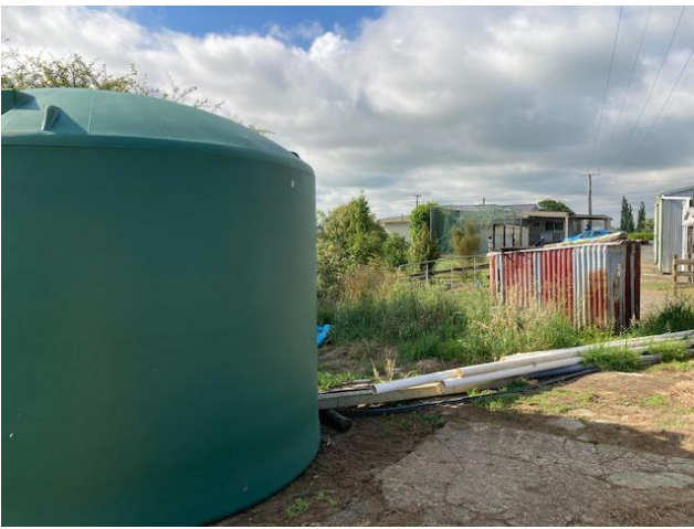
From tank to Club house where water will be collected from roof, piped to tank through filters & pumped to destinations.
