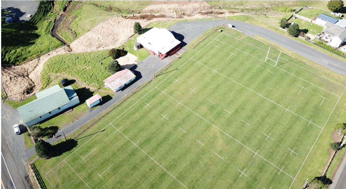
Te Kohanga carparking complete
