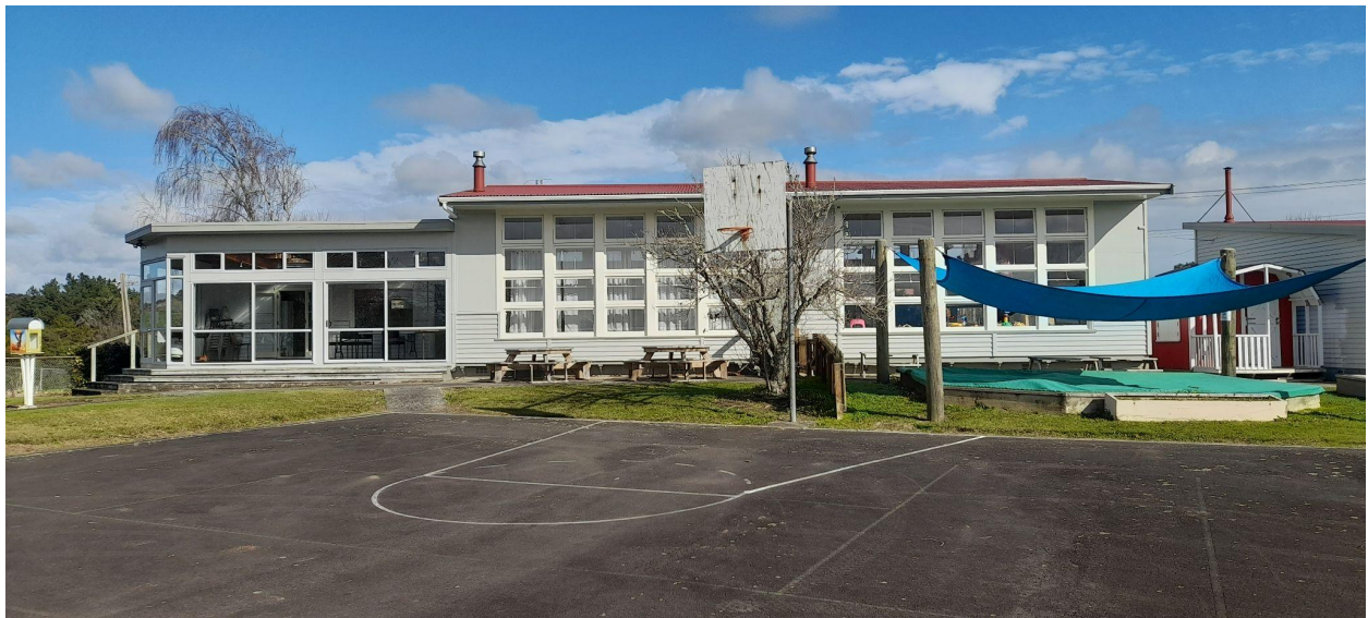
The main Community Centre Building
