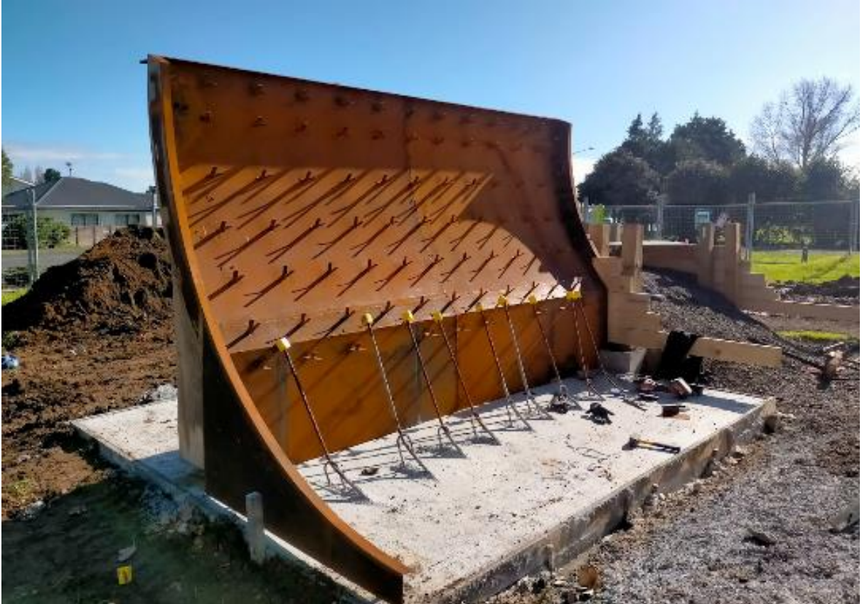
Tuakau Skatepark construction underway – Corten structure
