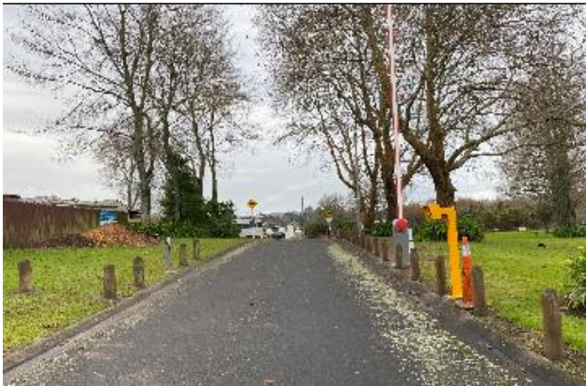
New camp entrance barrier arm
