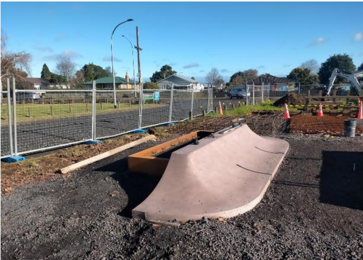
Tuakau Skatepark construction underway
