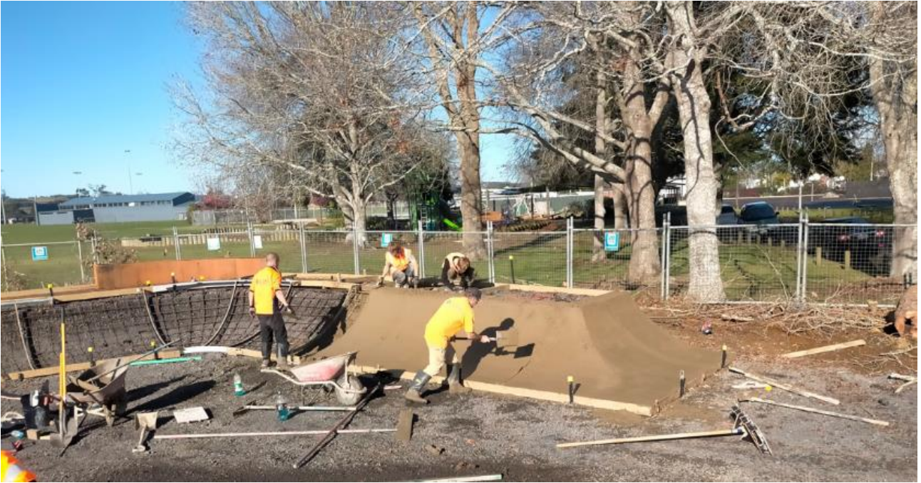
Concreting of features.
