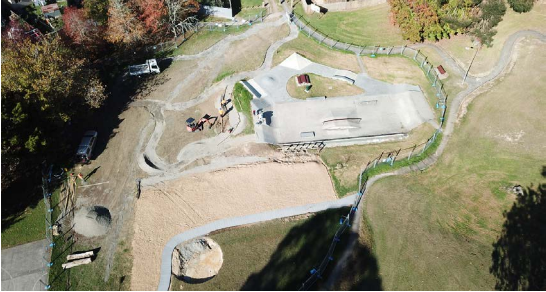
Works as at 13 May 2022
