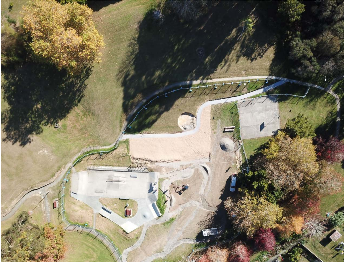
Works as at 13 May 2022
