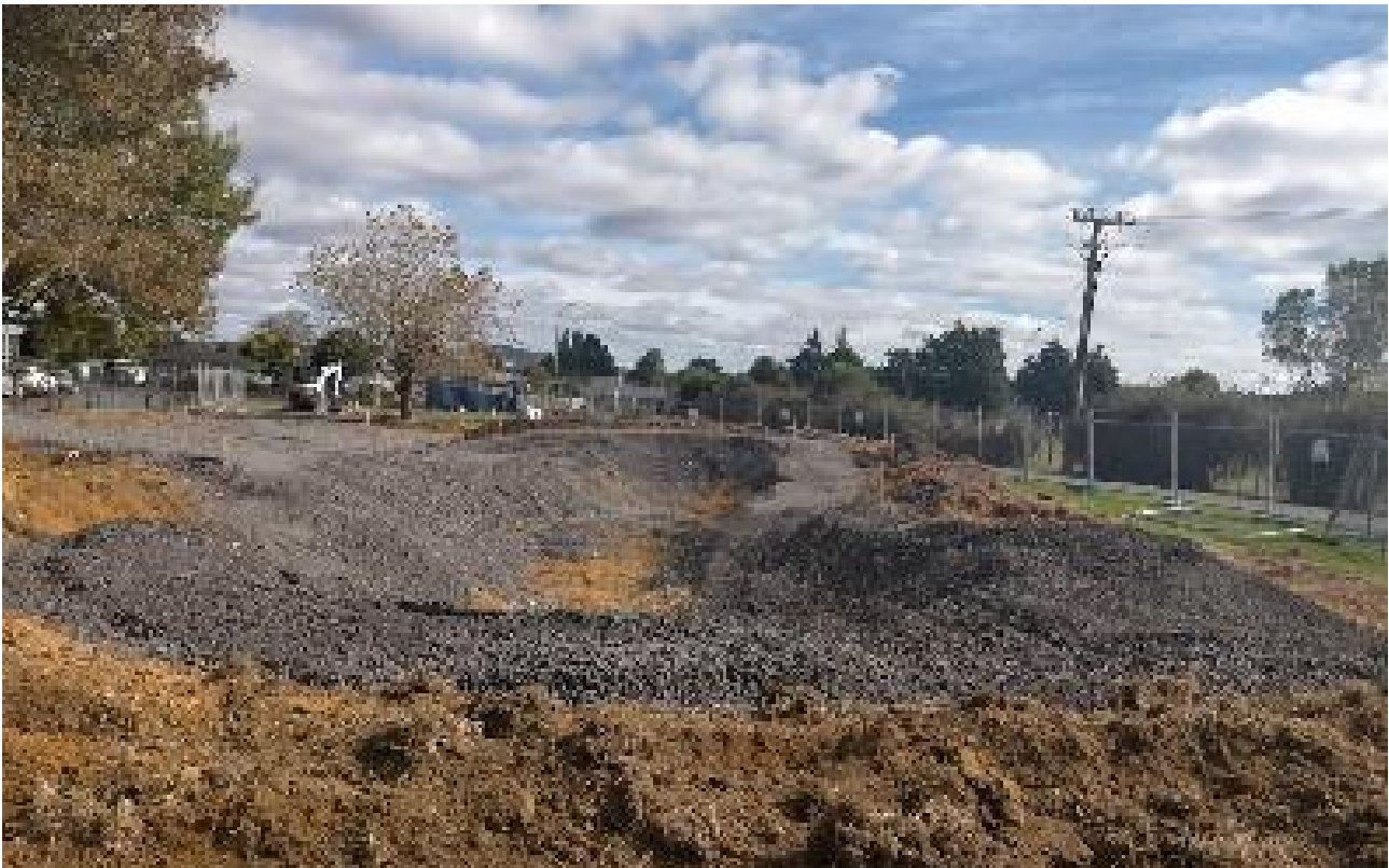
Tuakau Skatepark construction underway
