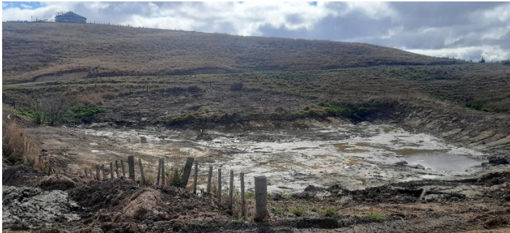
Whangamarino WTP – Pond 1 Sludge dried and cleared
