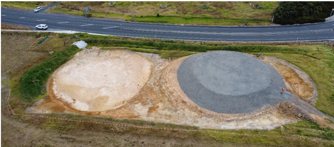
Te Kauwhata Reservoir- Preload for Reservoir 1
