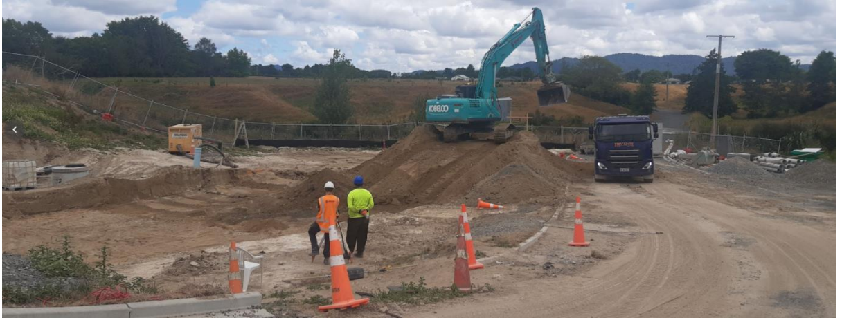
Earthworks at the new Horotiu Ports of Auckland Wastewater Pump Station
