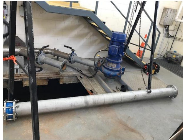
Galvanised pipe replacement
