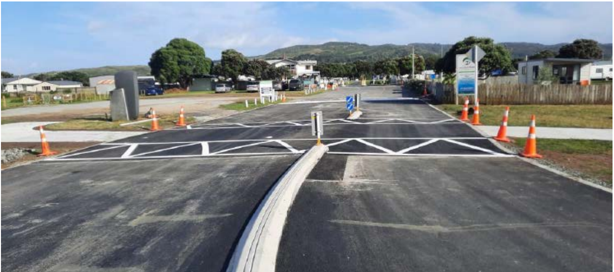
Campground entranceway works
