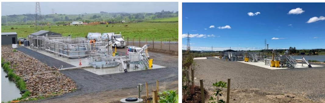
Meremere WWTP Upgrade – The process is now online
